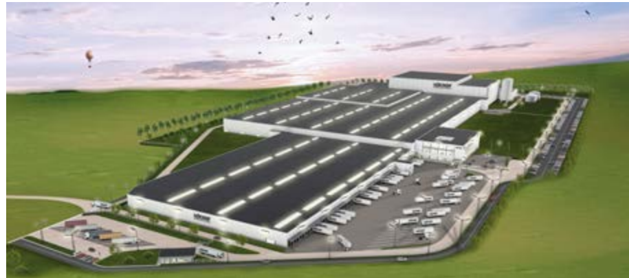
The ground-breaking ceremony commemorated the official start of construction. Commissioning is planned for autumn 2020.
