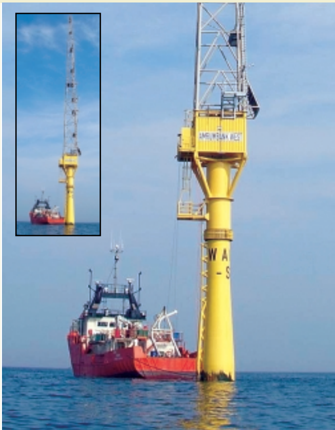
Abb. 1: Messmast Amrumbank West.
