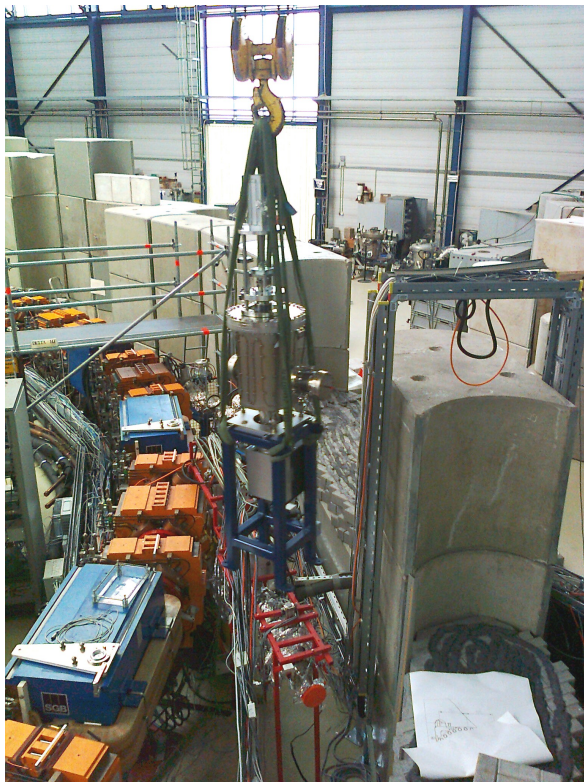
Fig. 1: Installation of the new beamshutter.
