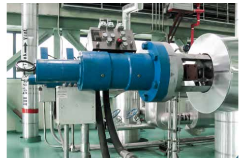
Hydraulic actuator for turbine bypass valve, with control function via proportional valve and quick opening function with three-way safety release.
