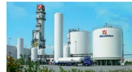
In its own air separation plants, such as here in Hörstel near Osnabrück, the Westfalen Group generates the air gases nitrogen, oxygen and argon.
