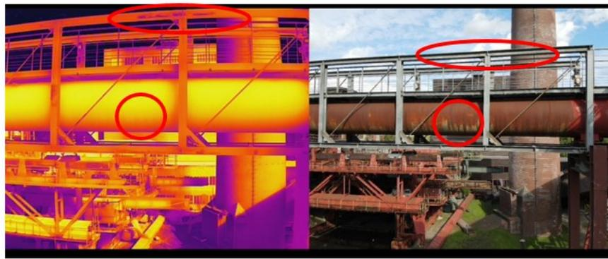
**Fig. 13.** Different views using RGB or thermal images. Different types of damages can be seen in each spectral band.
