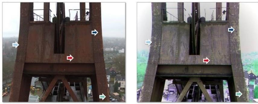
**Fig. 14.** Like in Fig. 18 multispectral images can detect plant cover like mosses and lichens.
